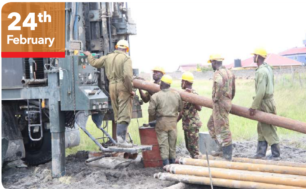
Kenya Defence Forces (KDF) Engineers' Water Drilling Squadron, sinks a borehole at Thika Landless.
