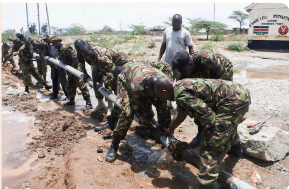
KDF troops from Engineers Brigade repair Archers Post-Larisoro main water supply line to restore water supply to residents in the town and its environs.
